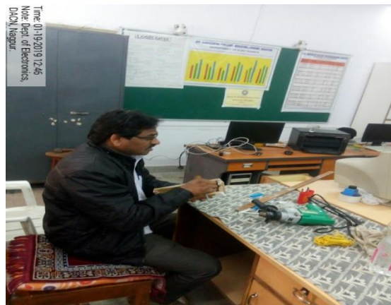
Shri Ram Ghode installing the Electrical board
